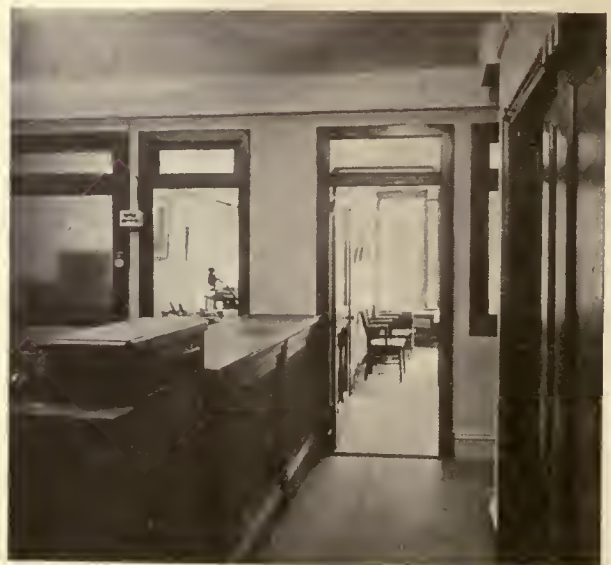
INTERIOR VIEW OF OFFICES
